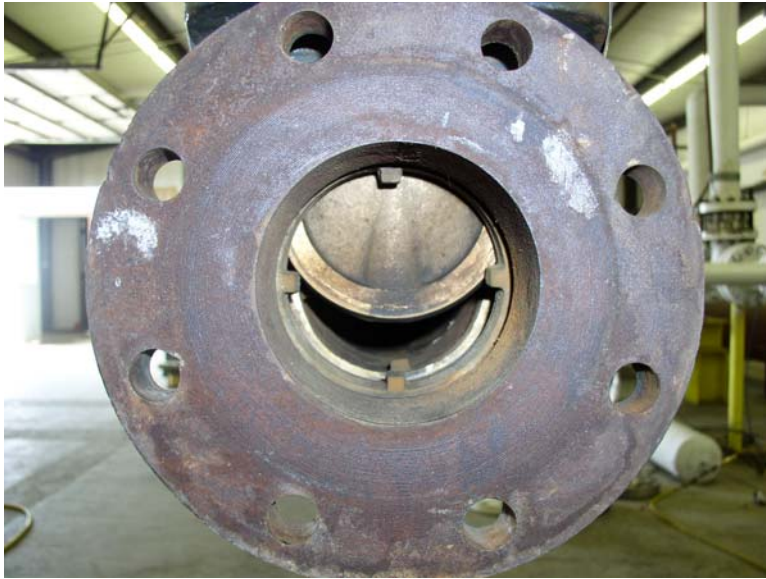
Fig 6. Half-Open Gate Valve
