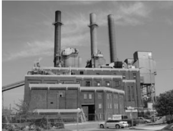
Fig 1: C.C. Perry K Steam Plant, Indianapolis
